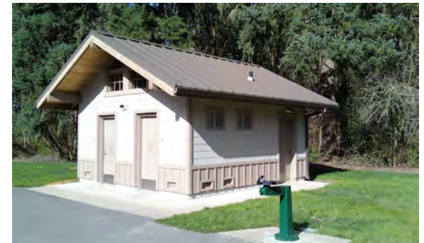
Simple auxiliary building with restrooms.
