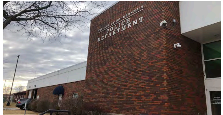
Police Station at 700 Main Street NW (Northeast Facade)
